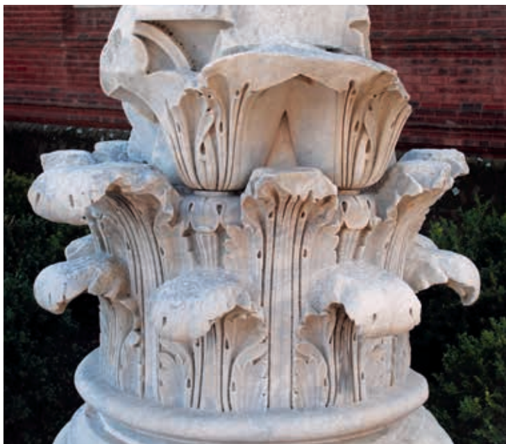
Since an 1895 fire destroyed the majority of the building, the architects and stone fabricators only had partial columns and fragments to work off of, as well as a couple of old photos. To begin, three-dimensional digital scans of a capital base and three smaller upper capital fragments of existing 1823 capitals were taken, creating a one-quarter-round composite marble and clay model. Photos courtesy of JGWA
