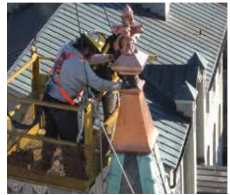
Replacement of copper narthex spire.
