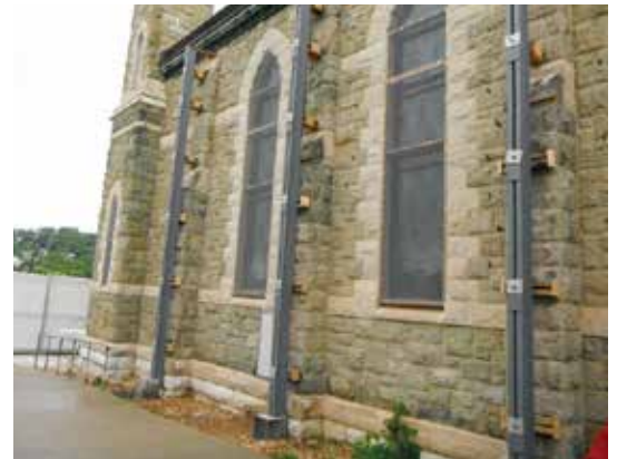
External strengthening buttress.
